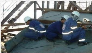
Cutting & Grinding Work
